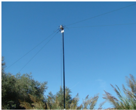
Fig.4 Configuration of the NVIS antenna
